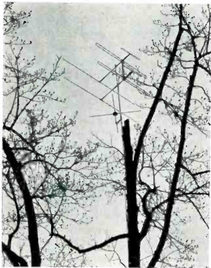
Figure 7 Three-top installation of a stacked array. 4 Turnstile antenna below the TV stack was installed to improve FM reception.
