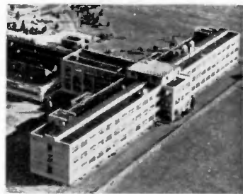
RCA Laboratories at Princeton, N. J., one of the world's centers of radio and electronic research. • When in New York City, see the radio-electronic wonders on display at RCA EXHIBITION HALL, 36 West 49th Street. Free admission. Radio Corporation of America, Radio City, New York 20.
