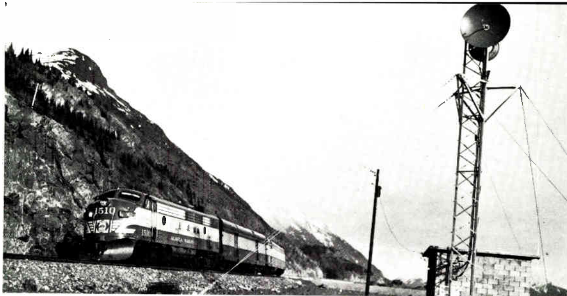
Microwave installation serving Alaskan RR System (Motorola).
