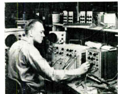
Testing Data Handling
