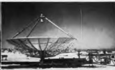
The antenna assembled but not erected.
