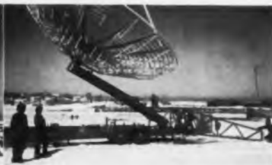
The antenna partially erected.
