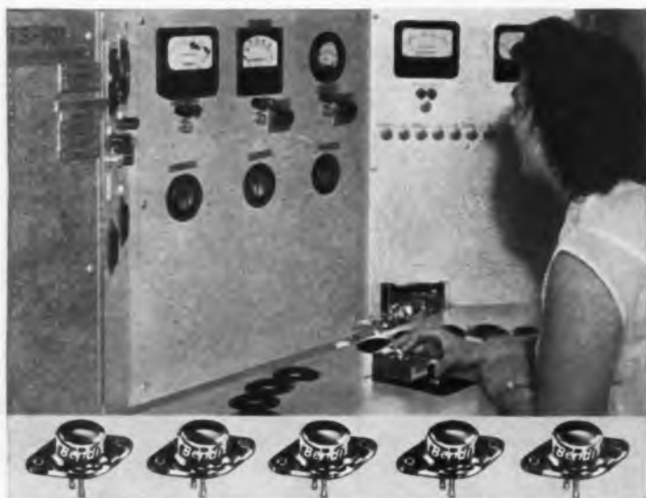
100% specification testing assures transistor rating.
