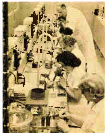
Fig. 23 (below): Peering through microscopes, these women are assembling delicate silicon transistors. Line foreman is checking work at one of the stations.
