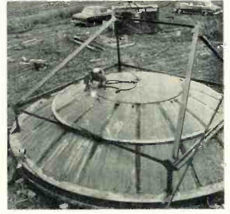
Fig. 4: Frame attaches to stiffening rings
