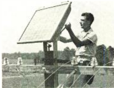
Telephone lineman adjusts solar battery
