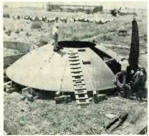
Fig. 2: Last reflector plate being positioned
