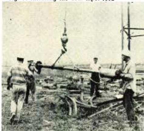
Fig. 5: Installing the dual input feed
