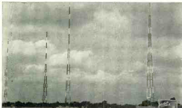
WKBN—Truscon Self-Supporting Directional Towers 350-Feet Tall
