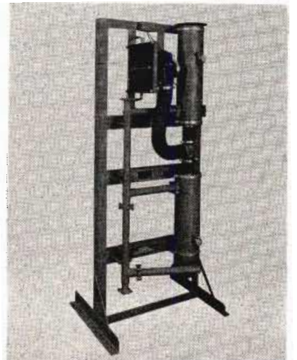
Fig. 11: Photograph of television diplexer unit
