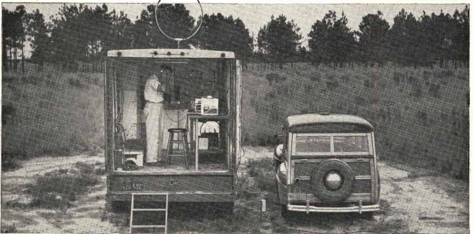
Thunder hunting equipment on location near Madison, Florida. Loop antenna on truck picks up static. The engineer in top picture is watching the indication of a circuit which registers how often the static exceeds a given level.
