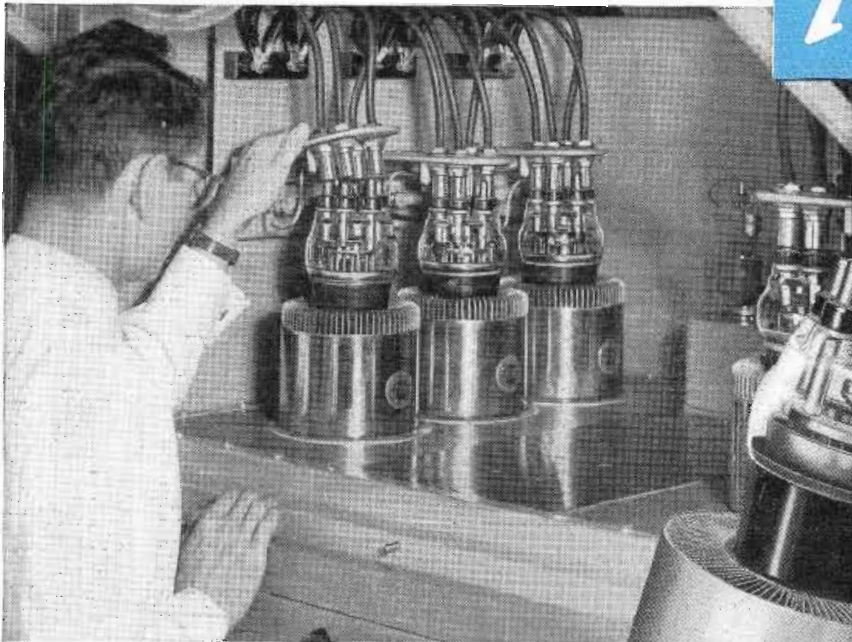
Installation of Federal F-8C25 power triodes in modulator tube compartment of 207B-1 transmitter.
