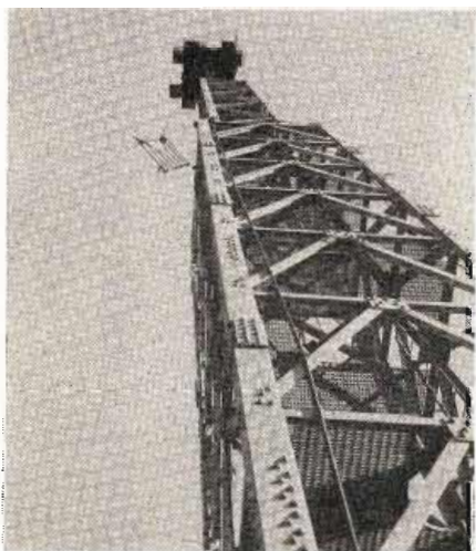
Steelwork as seen from tower base
