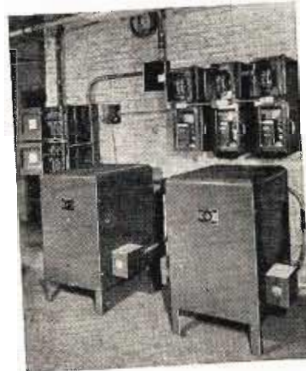
Elevator rectification — 3 bank power supply and regenerative braking equipment employing Seletron rectifiers, built for Clinton Realty Co., Chicago, by Ther Electric & Machine Works.
