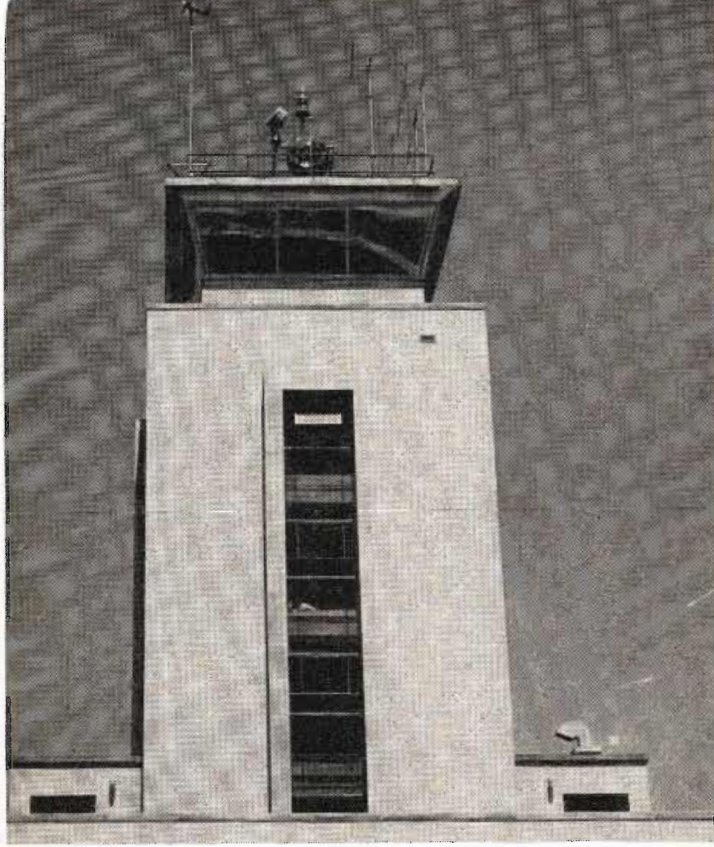
Fig. 1: Typical CAA communications and control tower shows multiplicity of transmitting and receiving VHF antennas
