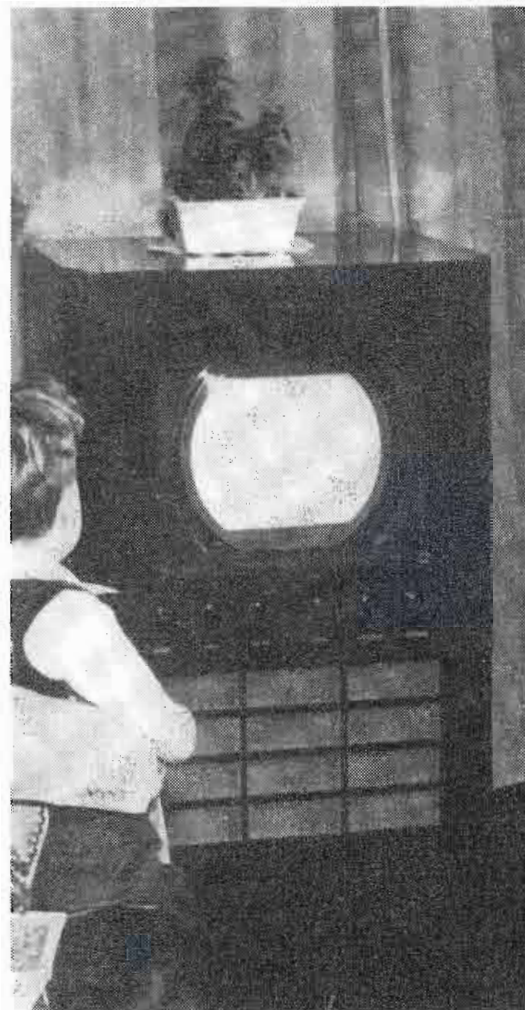
All-electronic RCA color-TV receiver. Color tube has 600,000 phosphor dots
