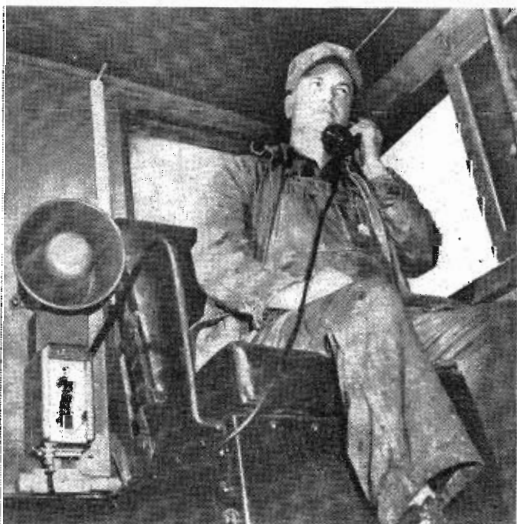
Fig. 1. Freight train conductor in caboose communicating with engineer in diesel loco over a mile away at head end of train.
