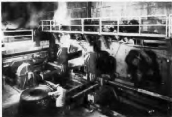
An employee at the new 44-inch semi-continuous hot strip rolling mill marks identification on a coil of strip steel after it emerges from the down coilers. High uniformity results from automation.
