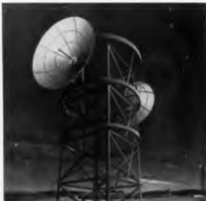
Guyed tower was designed and built by Blaw-Knox to meet the needs of a southern microwave system.
