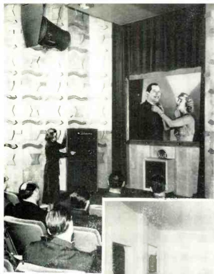
Fig. 1: (Above) RCA TLS-87 equipment projects life-size pictures, 6 ft. x 8 ft., from an out-of-the-way ceiling installation. (Right) Lounge at Perth Amboy New Majestic Theater has TLS-86 unit installed as moveable type console
