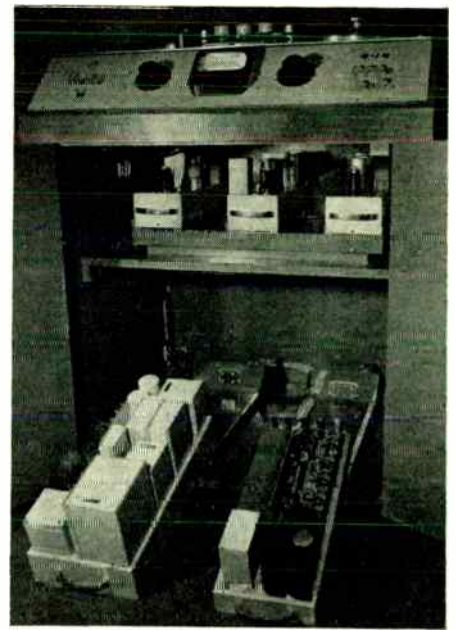
Fig. 3: Interior view of complete equipment shows unitized construction used throughout to speed and ease any required maintenance
