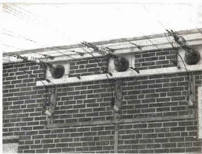
Left above is shown the base of the center tower used for daytime operation with the transmission line and quarter-wave shunt line used for tower lights and sampling line isolation. Right is a view of the RF transmission line showing lightning protection
