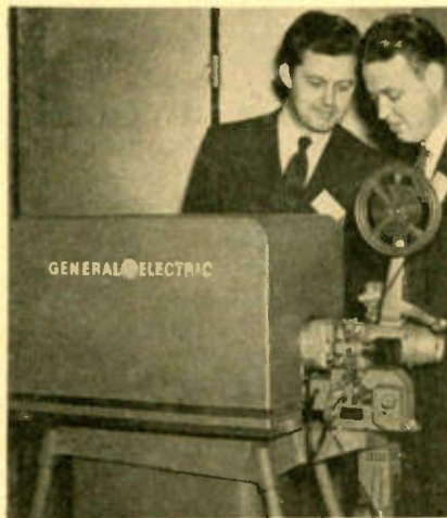
Eliminating the shutter, GE's pulsed light film projector is electronically synchronized
