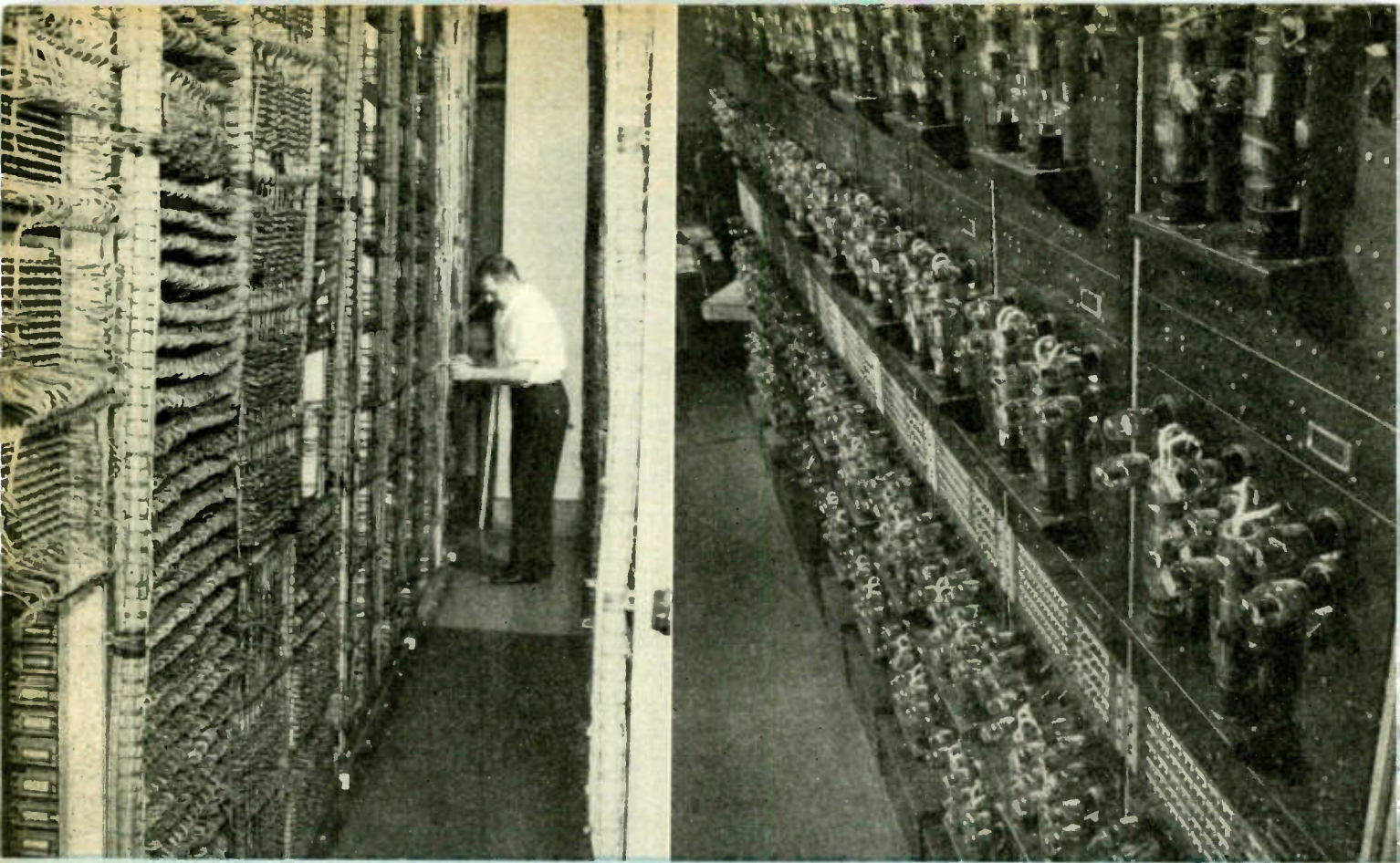
Behind the scenes view of some of the 2,000 tubes, 200 miles of wire, thousands of relays and switching equipment and 150 motors used
