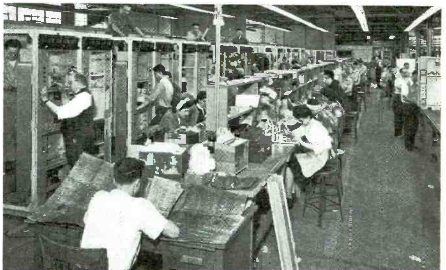
General view in the Newark (N. J.) plant of Federal Telephone and Radio Corp.
