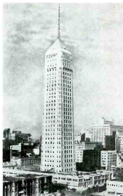
Foshay Tower (Minneapolis) topped by 8-element square loop FM antenna, manufactured by Federal Tel and R Corp., for 3 kw radio station WTCN
