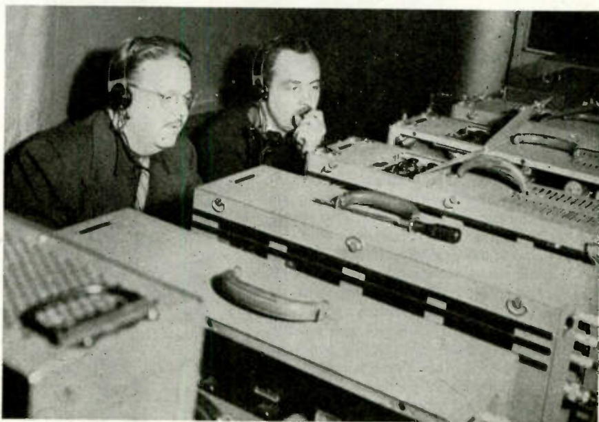
This is part of the extensive monitoring equipment used by NBC engineers and technicians on remote pickups for television, this particular installation being one that is used frequently in broadcasting Madison Square Garden sports events. This is the "suit-case" type of equipment
