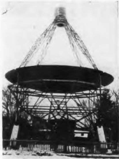
Fig. 1—Mirror-cavity device for collecting cosmic static
