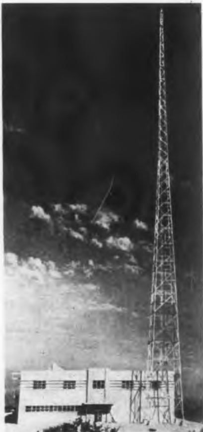
W6XAO's radiator is atop a 200-foot tower on Mt. Lee, elevation of which is 1700 feet
