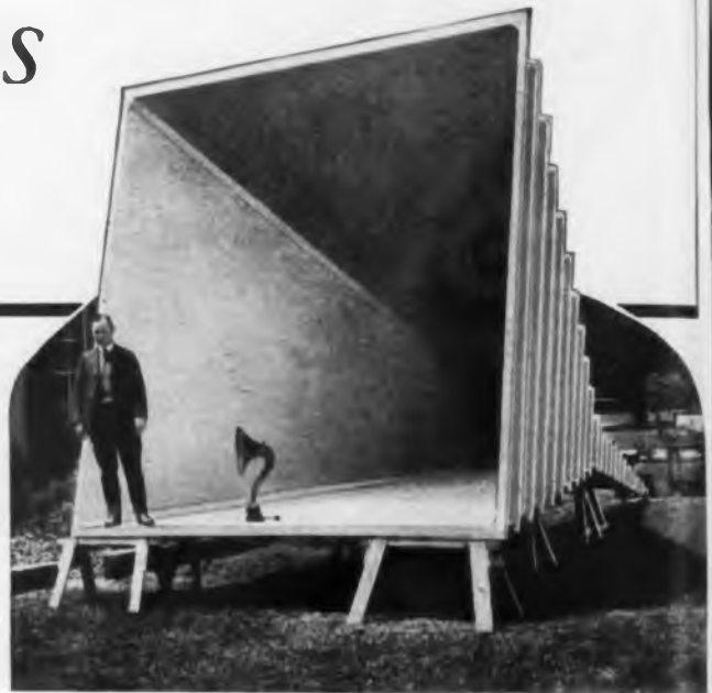
Largest loud speaker ever built—heard 9 miles. Built for Idora Amusement Park, Oakland, Cal., in 1922. Standing in the speaker is E. S. Pridham, now a vice-president, one of the founders of Magnavox, and co-inventor of the electro-dynamic speaker.
