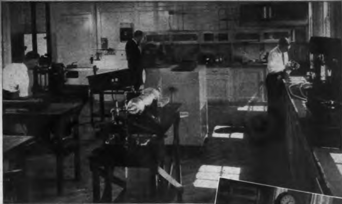
Section of Burndy's test laboratory
