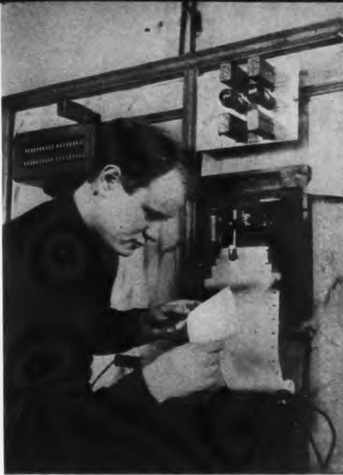
Russian designed and built telemetering-recording equipment used for control in dispatcher's office in a large oil field
