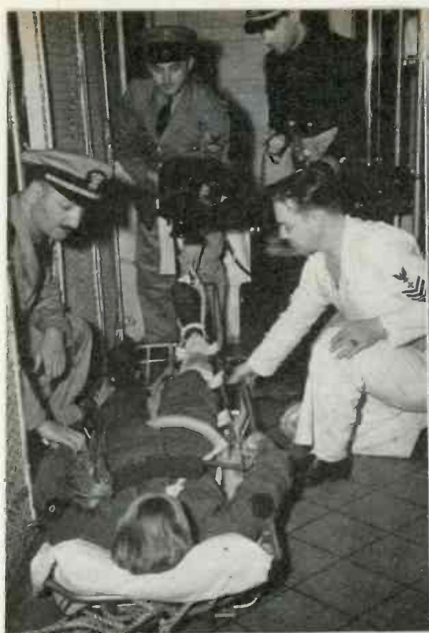
MOBILE-PORTABLE X-RAY —Packed in three cases, Mattern-Beeber unit can be assembled in 3 to 5 minutes without bolts or screws. Designed by Lieut. Commander W. N. Montgomery, Brooklyn Naval Medical Supply Depot, unit may be air or boat borne to isolated areas, and is used widely by Marines. Signal Corps photo shows Navy personnel X-raying leg of injured soldier enroute to Ireland
