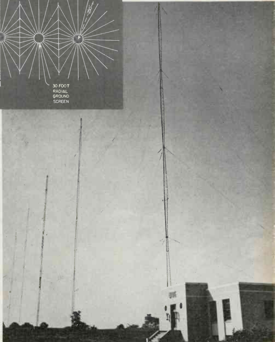
WIBG ground system and the five vertical radiators
