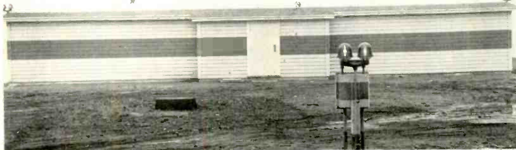
↑ "Inner marker" at LaGuardia airfield, located at start of landing runway. Projecting its radio energy upward, this marker gives pilot a final quick instrument check
