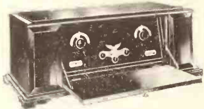
Model K2 Five Tube De Luxe Neutrodyne Receiver Cabinet finish: Adam Brown Mahogany. Genuine Duco Finish. Sloping Panel—Art Escutcheon. Battery Compartments. Width 15½ inches; height 13¼ inches; length 37½ inches. List Price $185. We recommend Power Tube.
