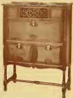
MODEL 121—RADIO CABINET. Loud Speaker Horn Built in with Removable 9 7/8 x 28 3/4 Mounting Board. Height, 46 in. Width, 35 in. Depth, 14 in.
