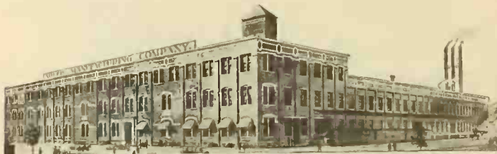
Where Adler-Royal Phonograph and Radio models are produced. These factories have always been devoted to the manufacture of musical instruments—their facilities for high quality cabinet work are also unexcelled.
