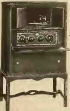
Pooley Radio-Phonograph ← Model 1500-R-3 Chinese Chipendale Style American Walnut or English Brown Mahogany, Duotone Finish Height 50", width 30", depth 18" Equipped with Atwater Kent 5-tube Model 20 Compact Set; built-in Pooley floating horn; Pooley phonograph in amplifying chamber. Price complete, less tubes and batteries—$295
