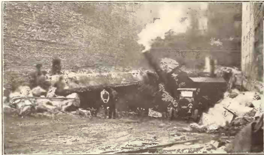
Breaking Ground for New Starr Co. Building
