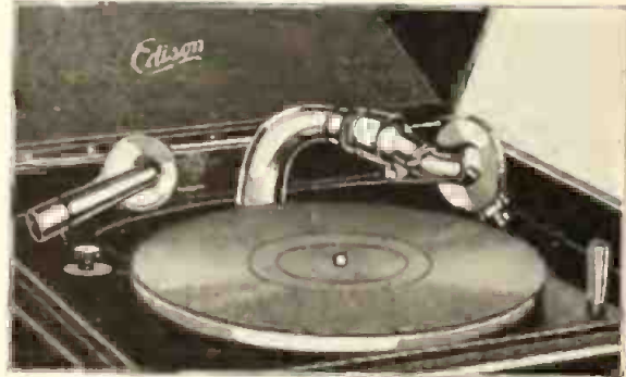
Showing Back View of Jewell Needle Equipment in Position for Playing Lateral Cut Records on Edison Phonograph
