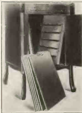
Showing shelves before setting into machine
