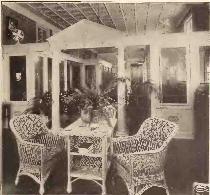
A Typical Van Veen Booth Installation
