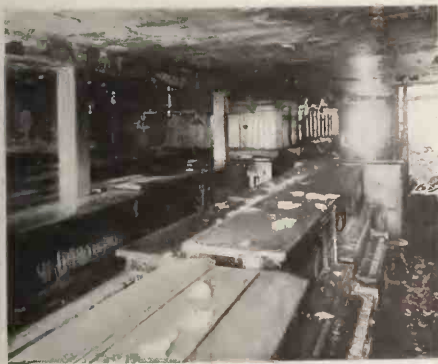
Another View After the Fire
