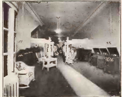
General View on Entering
