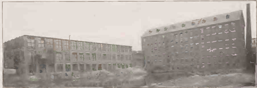
View of Part of the New Addition to the W. H. Bagshaw Plant.
