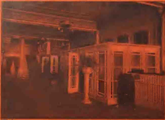
INSTALLATION FOR THE AEOLIAN CO.
