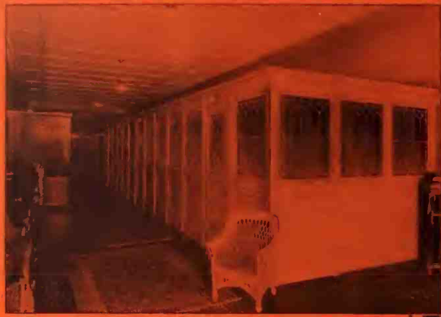
INSTALLATION FOR NEAL, CLARK & NEAL CO.
