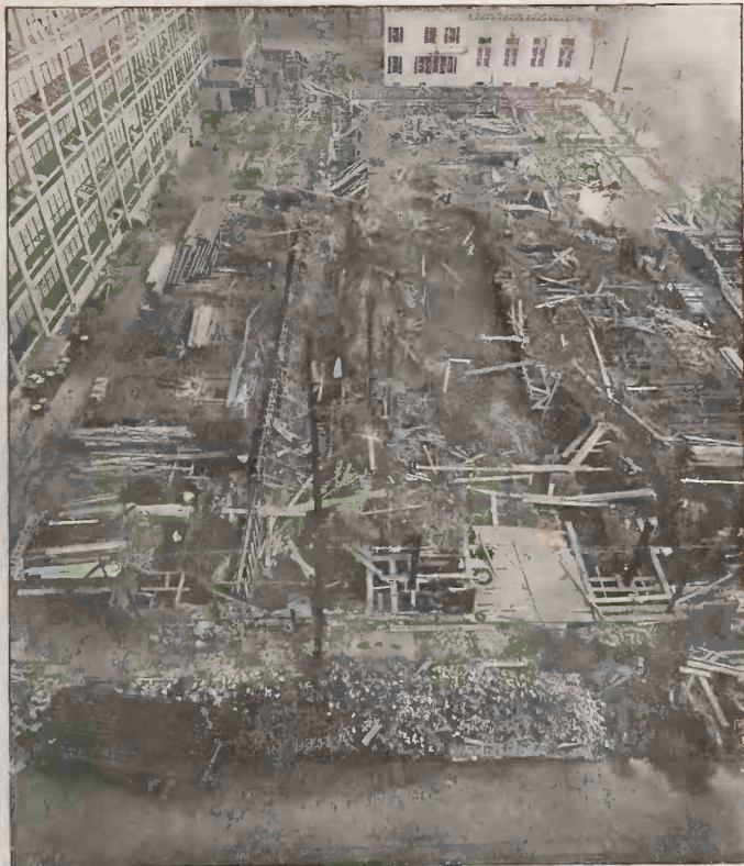
New Shipping Department Under Construction.
