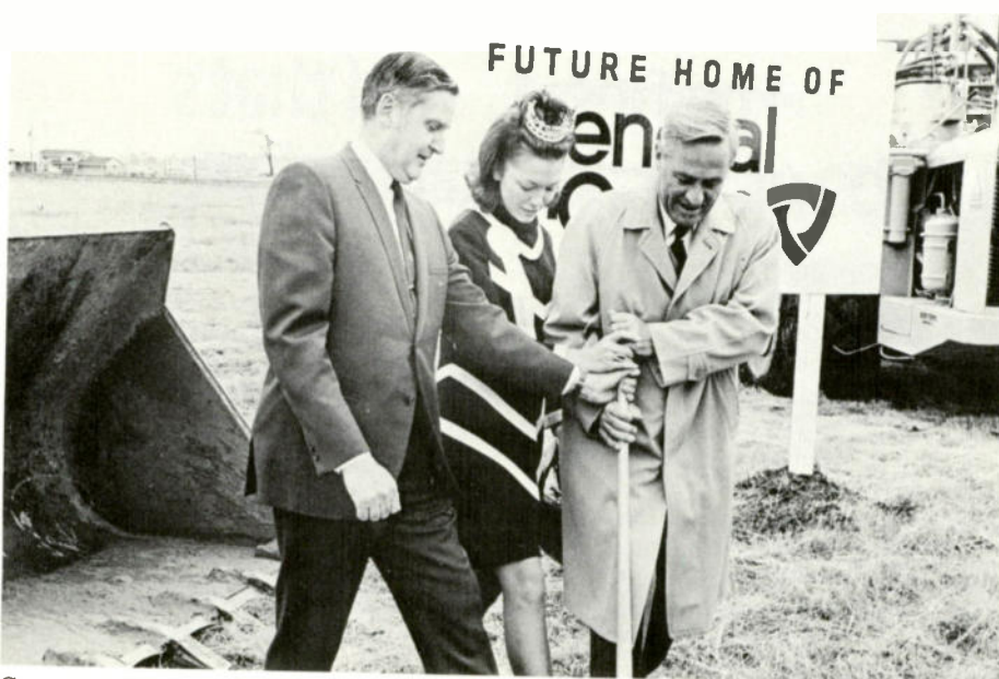
Governor John A. Love of Colorado (right) officiates at groundbreaking ceremonies signaling construction of a new General Cable Corporation manufacturing facility on a 25-acre site north of Denver in suburban Westminster. Assisting the governor is Robert J. Young, Jr., assistant general manager of the MOPECO division of General Cable, and pretty Sue Ann Gehrman, Miss Colorado. The 14,000-square-foot plant will also be used for storage of cable products.
