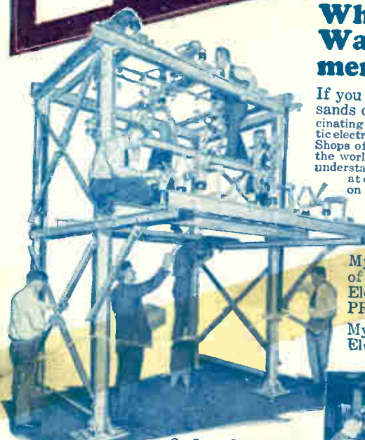
Students Constructing Outdoor Sub-Station at COYNE
