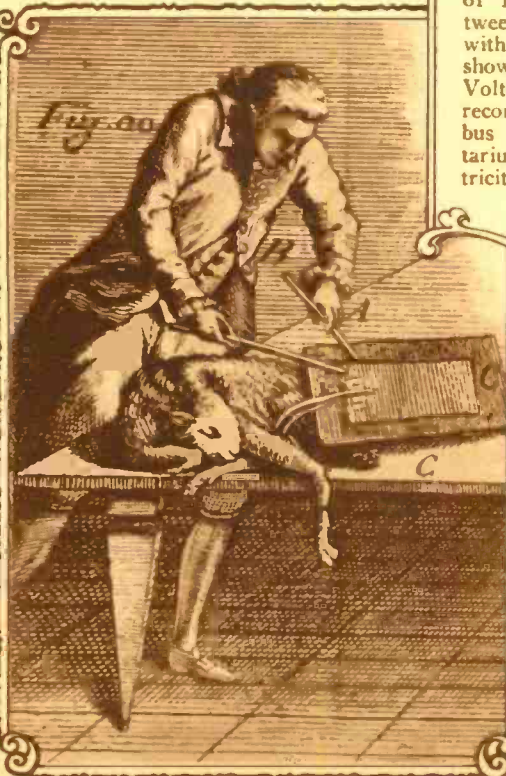
Most of Galvani's experiments were concerned with the effect of electrical currents on the muscles of frogs' legs. He contended that the muscular effect was due to electricity lodged in their legs.
