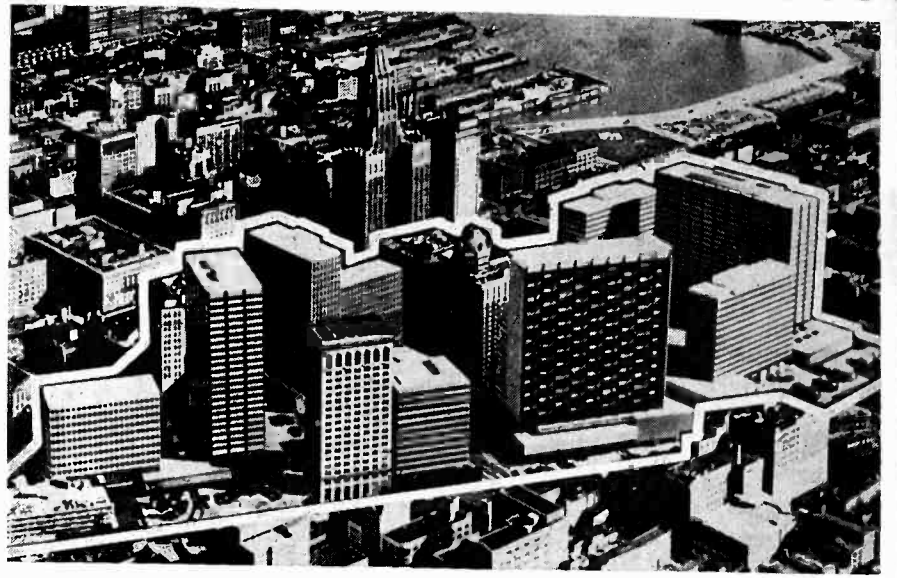
Baltimore, a City with its Face Toward the Future, has given concrete evidence of FAITH in an Ever-growing Economy by recently approving the proposed Charles Center, outlined above.
