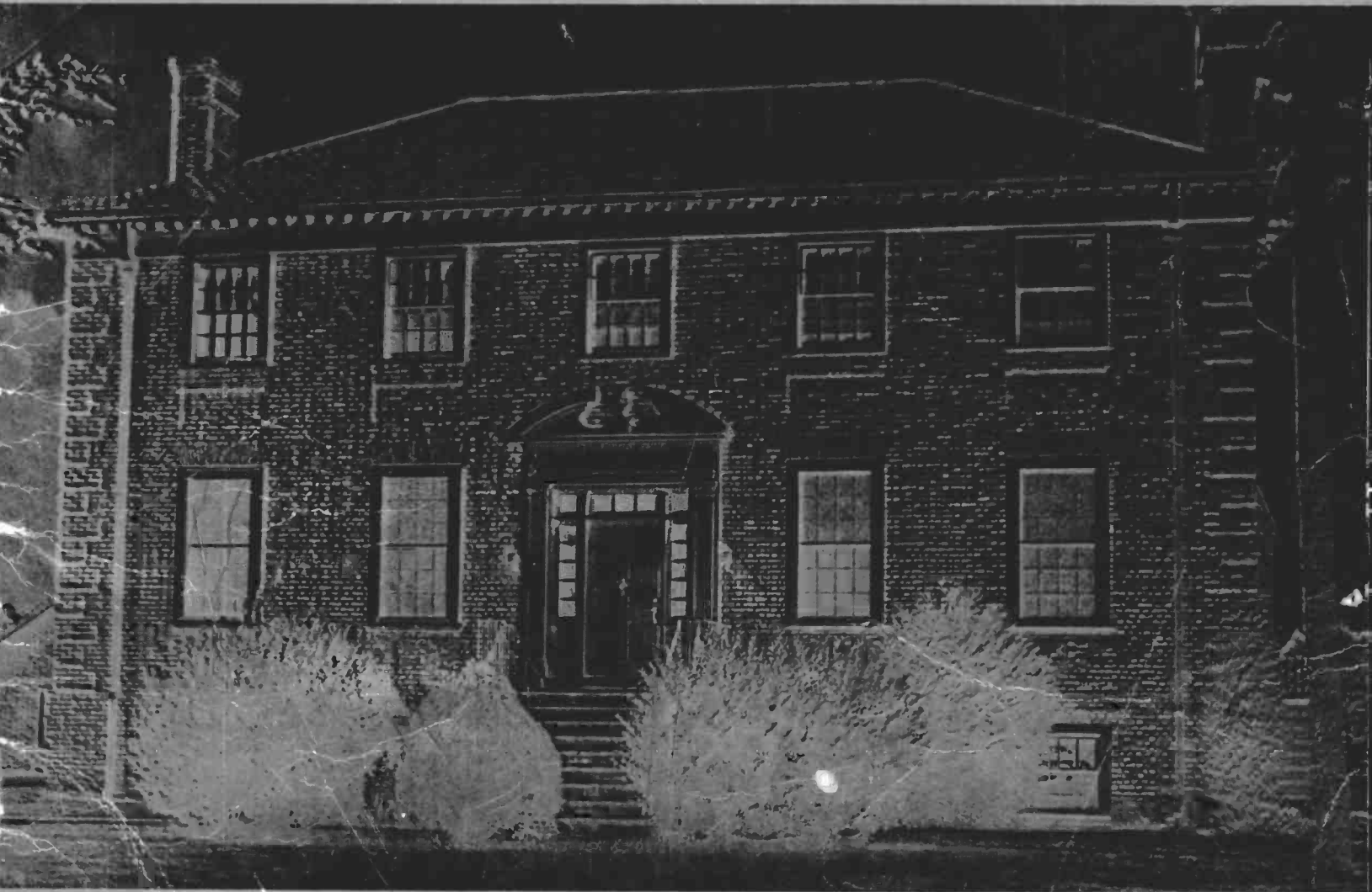
WRVA TRANSMITTER BUILDING AT EDGEWORTH - ON - THE - JAMES, NEAR VARINA
