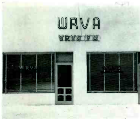
The WRVA and WRVC studios and WRVC transmitter are located at 2712 Colley Avenue in Norfolk. There we have installed the most modern equipment available to bring listeners the finest in AM and high fidelity FM broadcasts.
