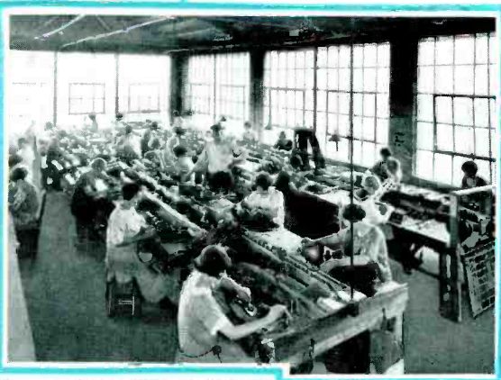
View showing a part of Neutrowound assembly department.
