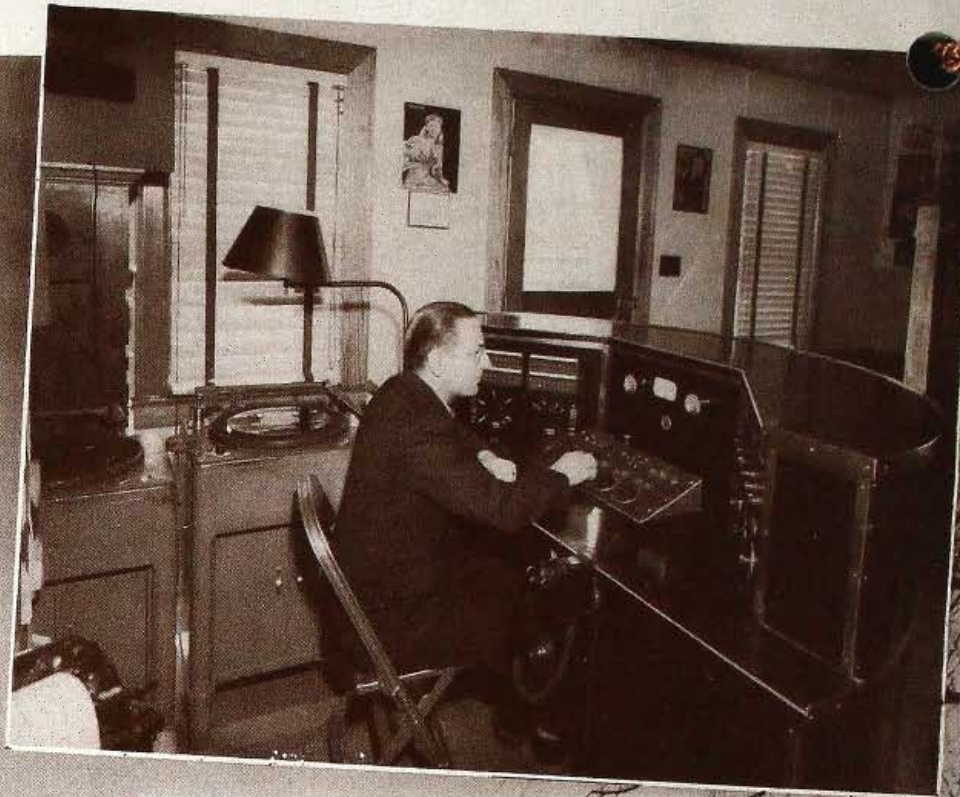
Chief Engineer JACK NAZAK at the transmitter controls.
