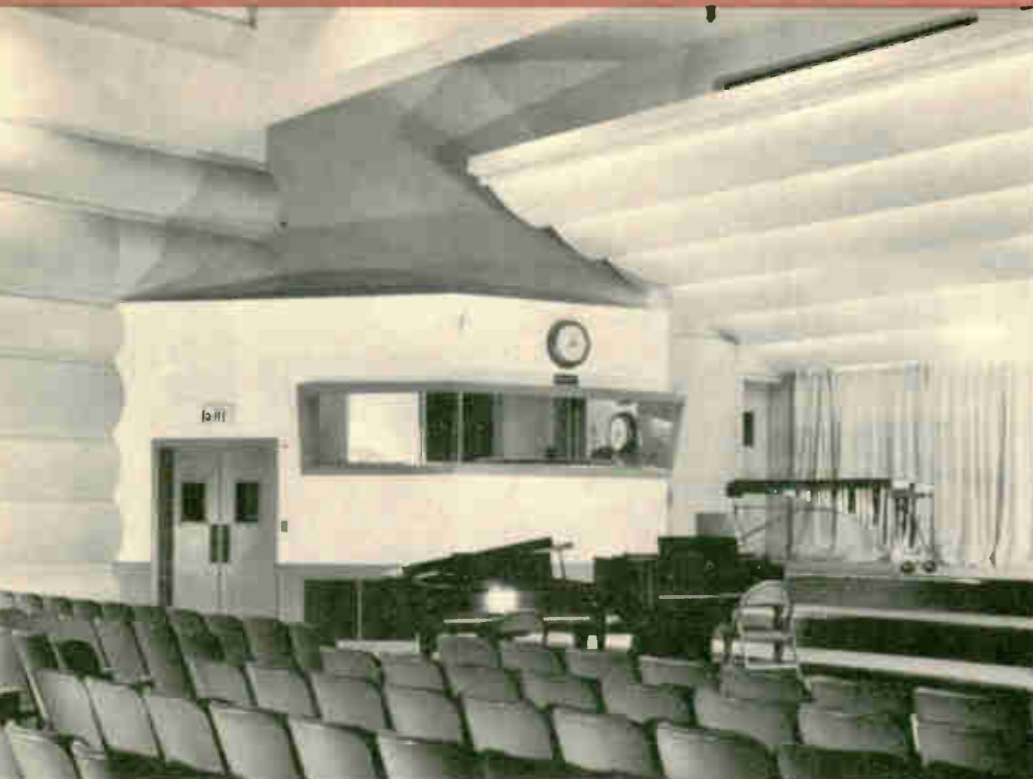
This is studio "B" which is the second largest at Crosley Square. This view shows the comfortably upholstered seats, the control room and the indirect stage lighting. Note the polycylindrical construction of the side wall for the utmost diffusion of sound.
