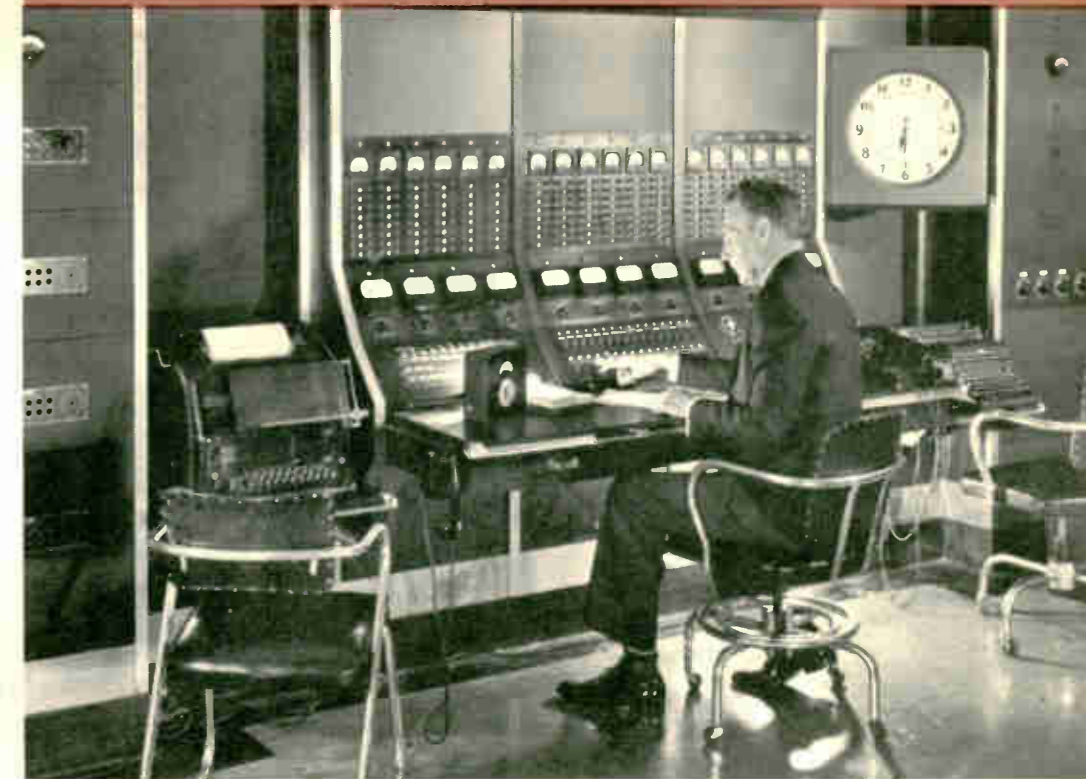
There is always an engineer on duty at this master control—the nerve center of Crosley Square. From the studios and the networks, programs travel by wire to this panel. From here they go by wire to the WLW transmitter 20 miles away at Mason, Ohio.
