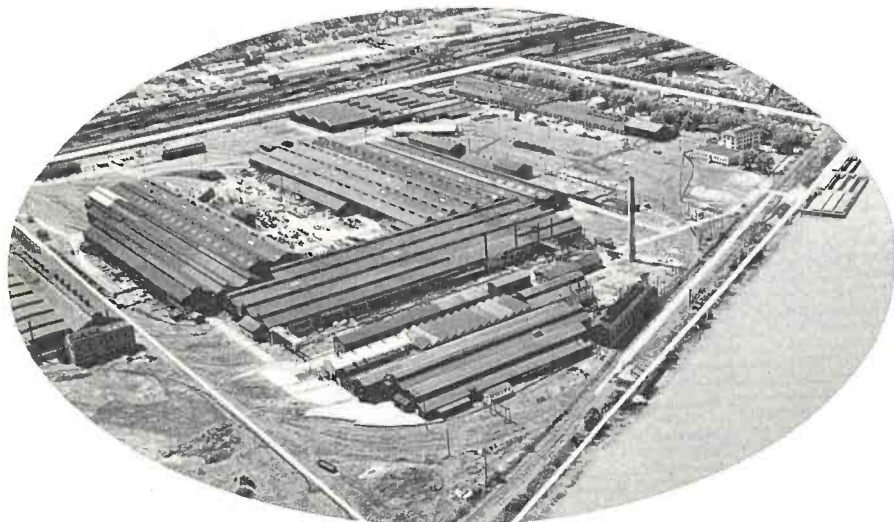
Site of the Pittsburgh District's new 103 acre River-Rail-Truck terminal.
