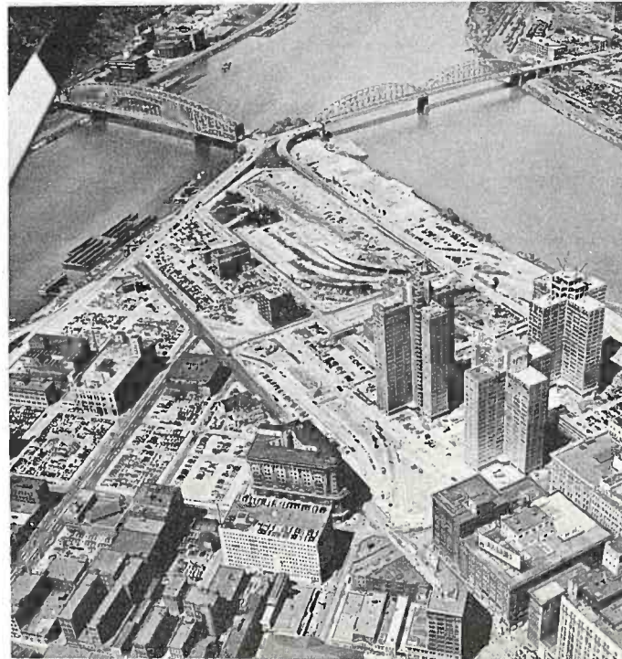
Rebuilding underway . . . three of the eight buildings to be constructed in Gateway Center are shown.
