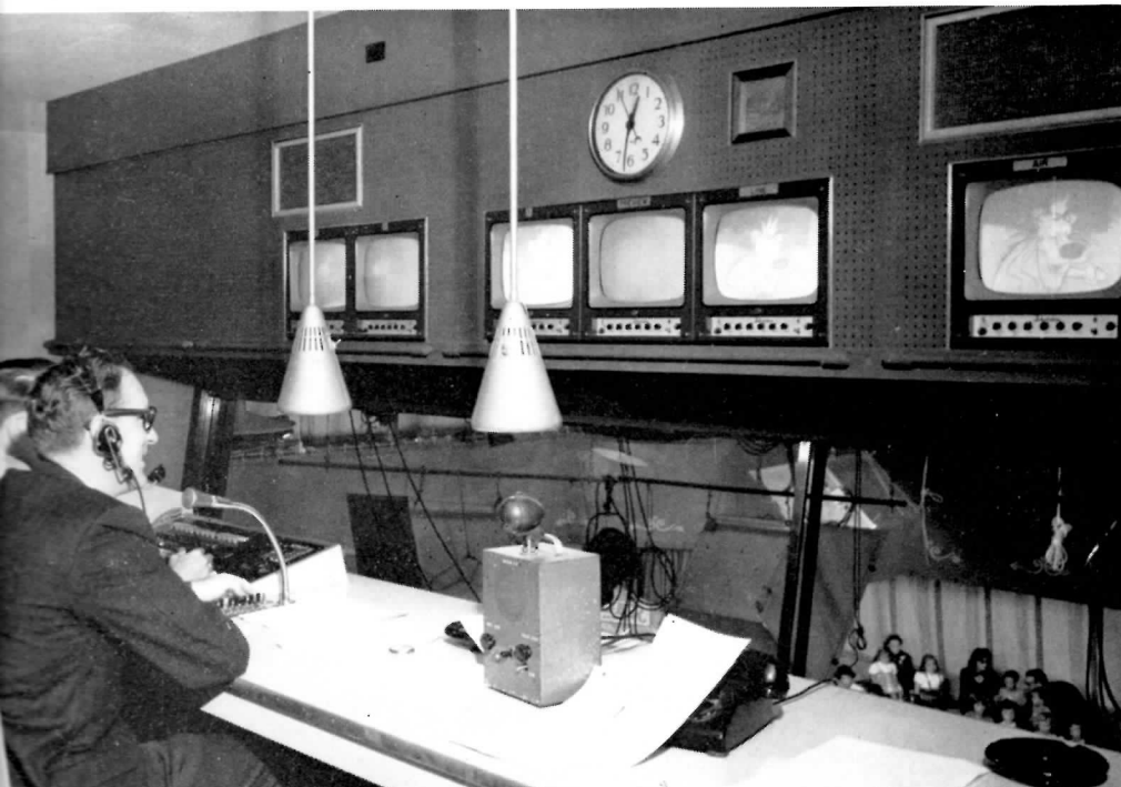
FIG. 13. Control room, 15 ft. above studio floor, gives good visual coverage of studio.
