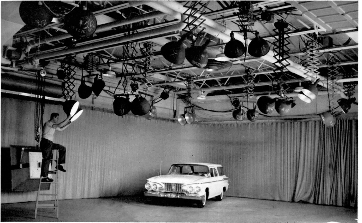
FIG. 20. Turntable in floor and studio facilities in corner of garage are suitable for automobile and agricultural commercials.
