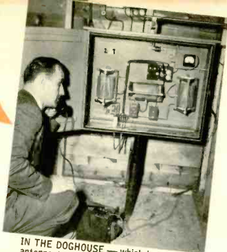
IN THE DOGHOUSE — which houses the antenna tuning equipment we see Chief Engineer Shimski making required tests.
