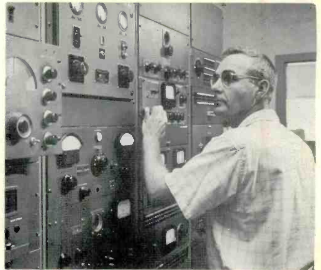
Transmitter Engineer Al Loehlien watches the dials on test panel to make certain WCCO Radio's signal is steady within one part in 830,000.
