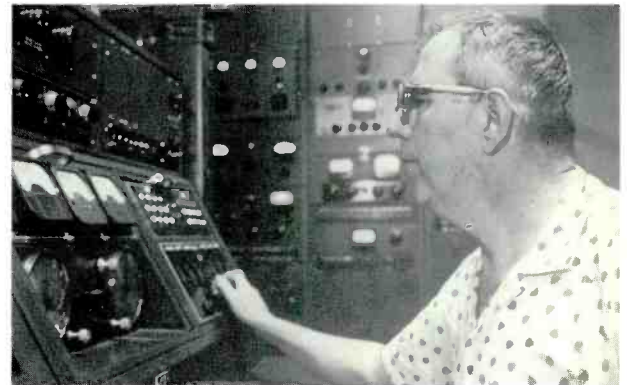
The man nobody ever sees — George Collier, in charge of the two 50,000 watt transmitters and short wave equipment and emergency installations in Coon Rapids, near Anoka, Minnesota.
