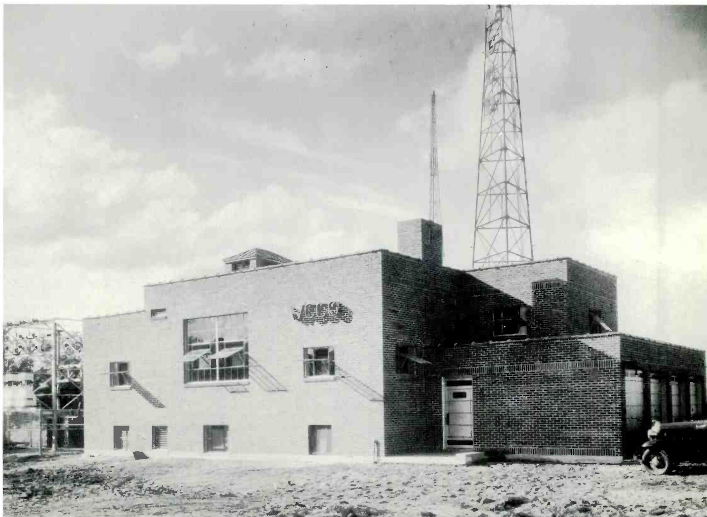
The expanded transmitter was completed in the summer of 1932. This building still houses the original equipment and an additional 50,000 watt transmitter and special emergency and remote broadcast communications apparatus.
