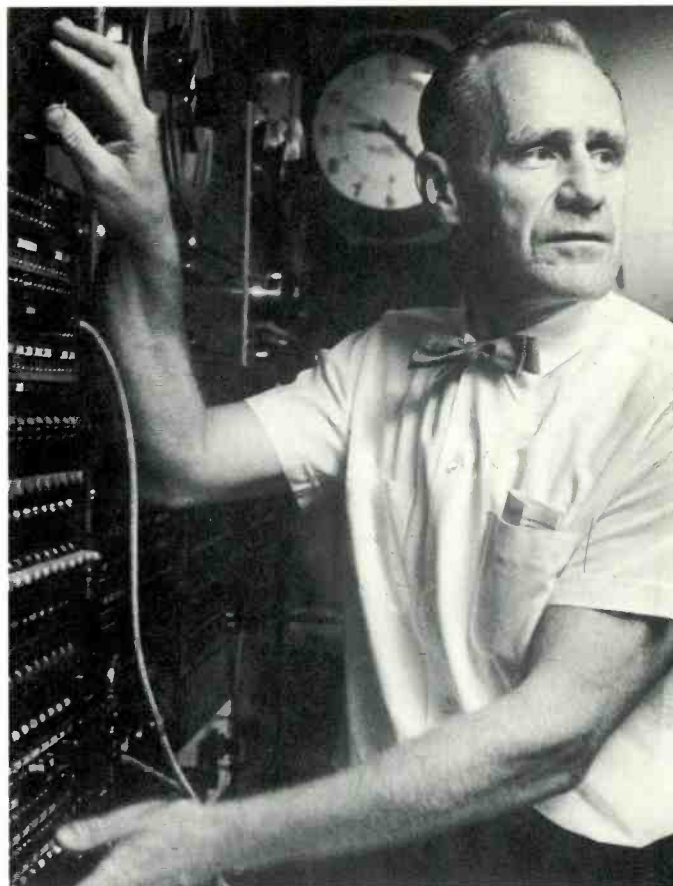
Studio engineer, Harland Gabrielson, works controls at the "patch panel." All WCCO Radio programs from home studios, CBS network and remote points come in and go to the transmitters through this panel. Typical programs are broadcasts of the Minnesota Twins, Vikings and Gophers, fed from here on WCCO network.
