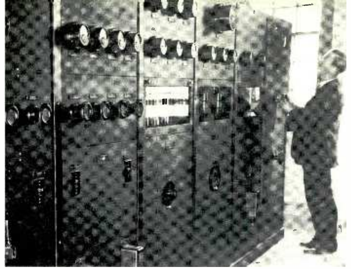
A WCCO engineer adjusted voltage at the control panel of the station's new 5,000-watt transmitter in 1925. This transmitter has an interesting history. It is the one that Twin Cities crystal set owners could not hear on the morning of the Coolidge inaugural, March 4, 1925, because it was too far out in the country. When WCCO's power was increased to 50,000 watts, this transmitter was sold to old WDGY, the Dr. George Young station. It was sold again in the late 1930's and recently was being used somewhere in South America.
