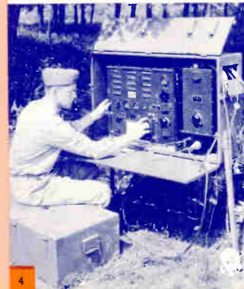
4 Close-up of Army Field transmitter.
