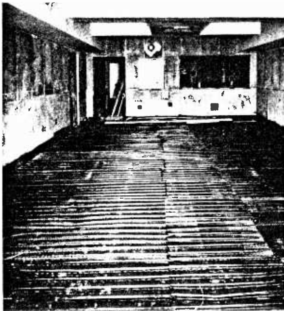
Figure 6. Wire mesh laid over black building paper, ready for concrete floor.
