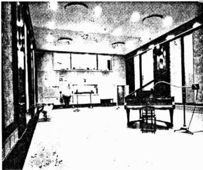
Figure 19. One of the 30' x 50' x 18' studios on the third floor, showing the sliding acoustical panels partially open.
