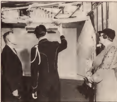
MR. AND MRS. MILLION (the I. V. Goodmans) of Ardmore, Pennsylvania are shown above having the studio construction exhibit in the air conditioning plant explained to them by Guide Bob Kennedy. Nice picture of Bob's back, isn't it?
