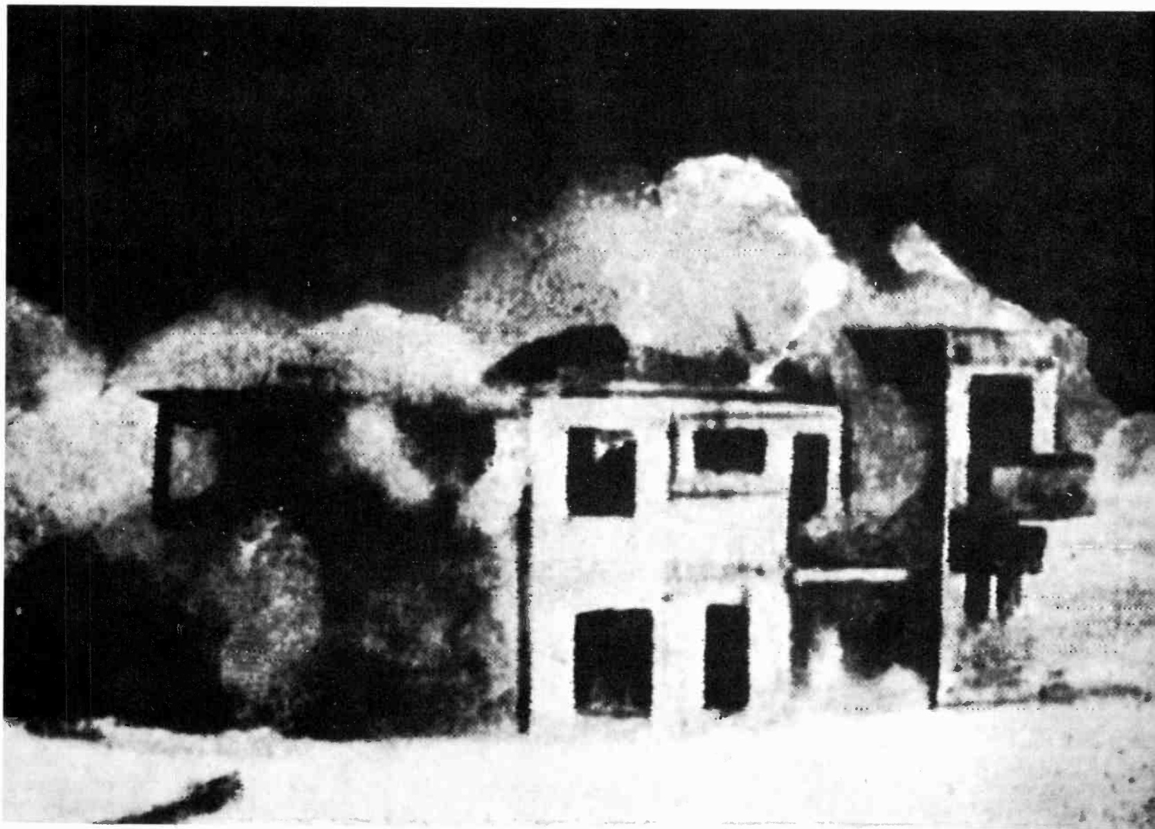
Atomic-blast films released by China in a forty-minute-long color film show a brick building being destroyed in the blast of what was believed to be the nation's third nuclear test. One thing was certain, though: Red China became a nuclear power years sooner than expected.
