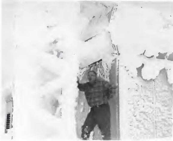
The weather at the summit of Mt. Ashland. . .7,500 feet high. . .becomes rather rugged during the winter, with ice and snow encasing the tower and wrapping around the building.
